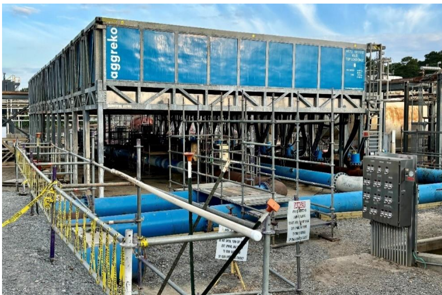
Figure 2 Individual Modular Design Allows for Interconnected Cooling Tower
