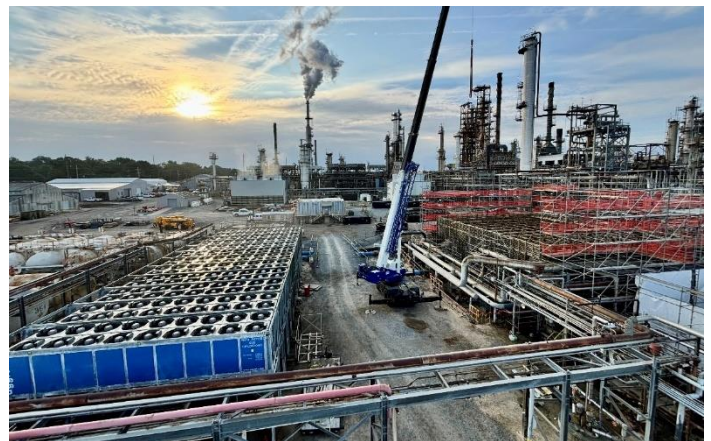
Figure 1 (12) Interconnected Modular Rental Towers for Demo & Construction of Replacement Cooling Tower.
